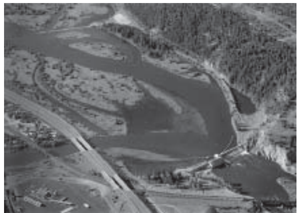
An aerial view of the Milltown Dam before its removal. Photo courtesy Clark Fork Coalition.
